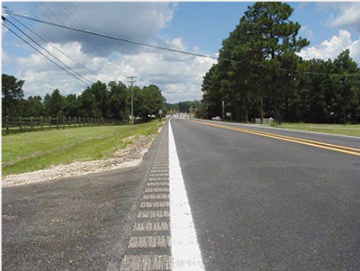
INSTALL SHOULDER RUMBLE STRIP
