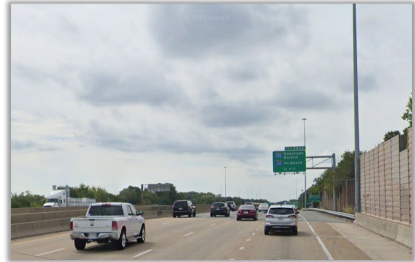
I-64 EASTBOUND NEAR I-264
