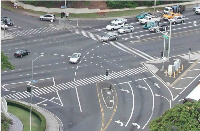
IMPROVE PAVEMENT MARKINGS
