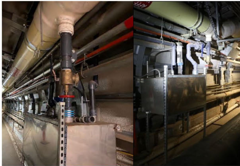
Final Installed Low Point Drain System with PVC Retention Line
