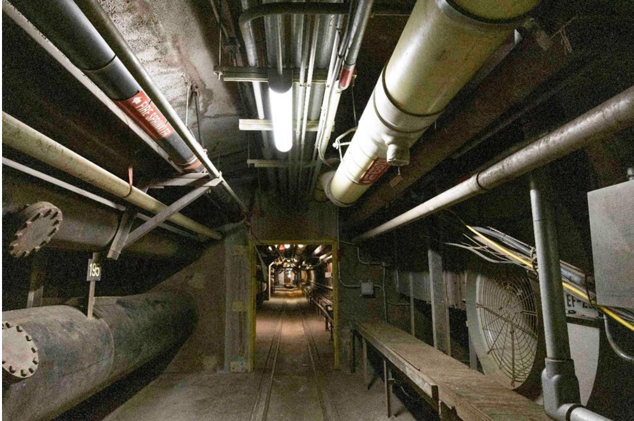
Lower Access Tunnel with AFFF retention line in top right (PVC pipe)
