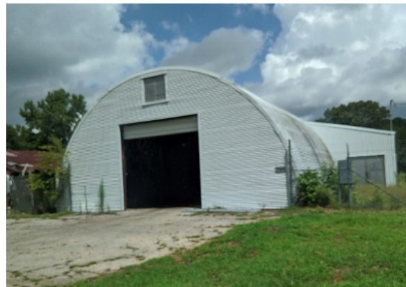
Grounds Maintenance Shed
