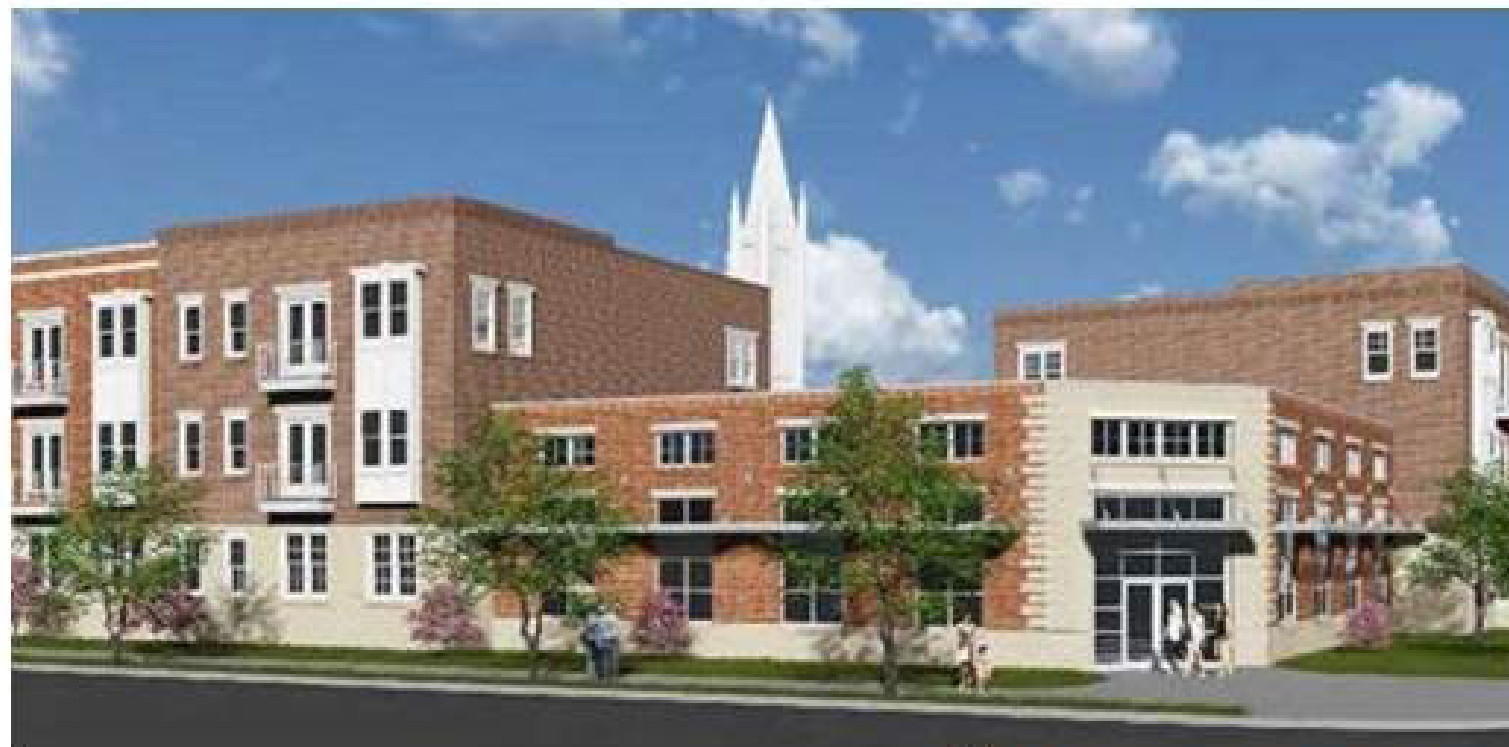
* St Paul's Apartments
